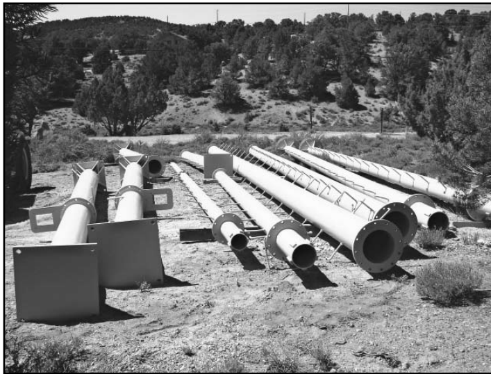
These two rotating towers, 120 feet and 190 feet, will be in the air this summer. The 120 footer will support 6/6/6/6 on 15, while the 195 foot tower will support 6/6/6/6 on 10 meters and 3/3 stacked OptiBeams on 80.
