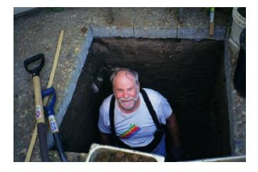
When I thought I couldn't dig any more, I built a big rebar cage, and hung it in the hole from some wooden forms. I had the hole inspected by the city, which gave me permission to pour concrete in... to fill up the hole I had just dug!
