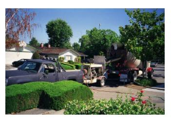
Next I bought a load of concrete, and hired a pump and a long hose, like the rig shown above. This was used to put 9000 pounds of concrete into my city-approved, XYL-approved hole in a bit under three minutes!
