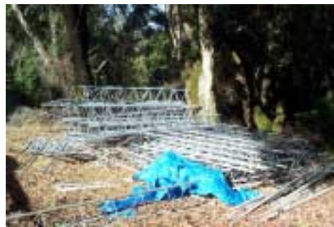
Tower sections...lots of tower sections
