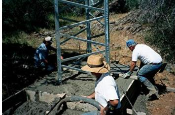
Topping off the tower rebar-ed into the rock. You can see a stream of concrete coming out of the hose.
