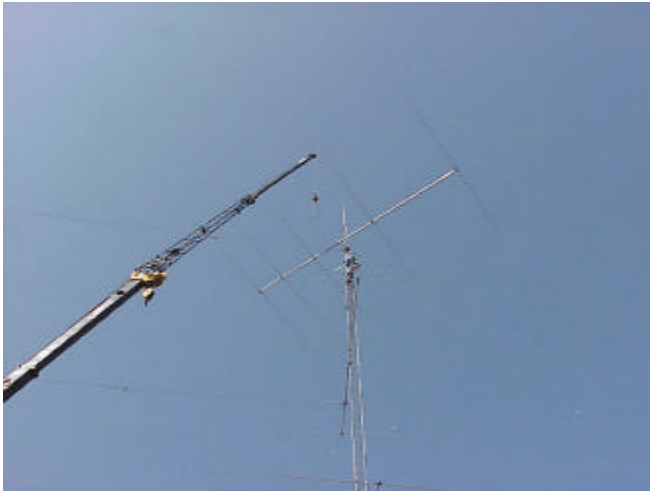
At WC6H, a 5 element KLM 20m Yagi and a 4 element KLM 40m Yagi were taken down to replace a bent mast. The crane is sure a good way to move things around up there!
