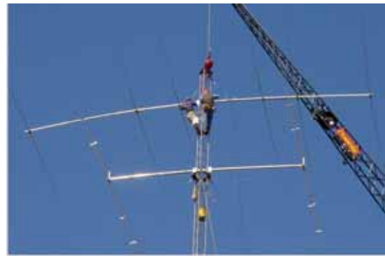
K7NV and W2GD install the top two antennas
