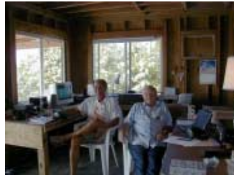
Bruce and Bob, W6CYX, do a CQWW, together, even before the walls had been insulated and covered with sheetrock.
