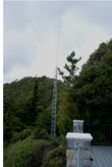
Al works 80 and 160 with the Hy Tower vertical that has been bolstered with heavy strapping to handle the brutal winds.
