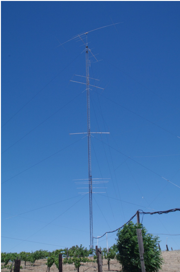
Figure 12. The completed tower shining in the California sun.
