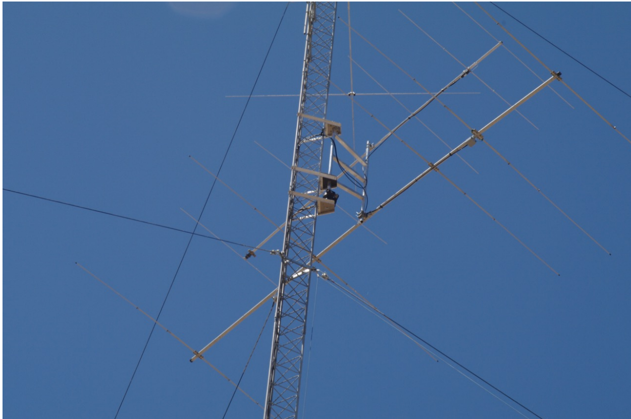
Figure 6. A swing-arm mount supporting two antennas. This one is fabricated from aluminum by Robin, K4IDC.
