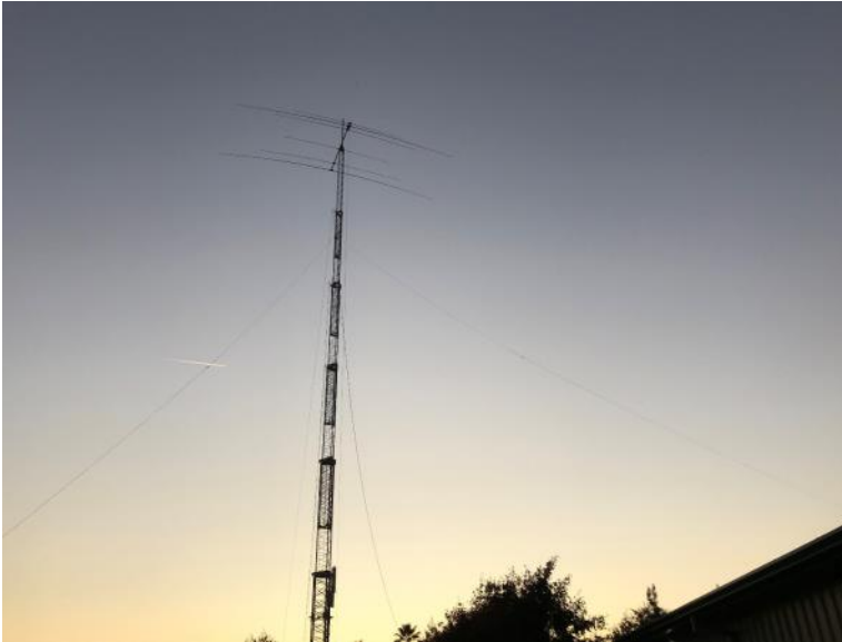
Figure 5. CQP 2019: NS6T antennas: 2-el Force12 C3S Yagi at 100ft., 40m Inv-Vee at 85ft., 80m Inv-Vee at 70ft. All supported by a US Tower portable tower trailer
