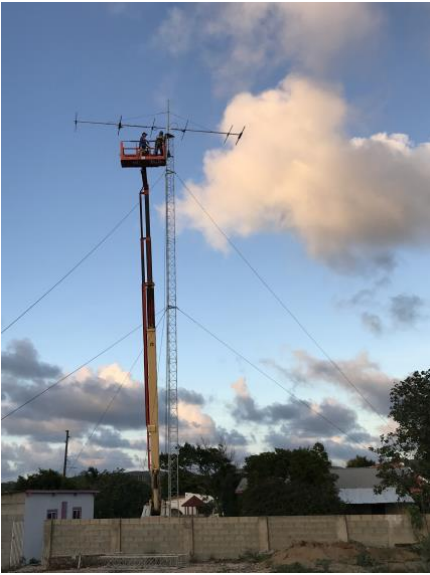
The 2040 being installed on the Rohn 45
