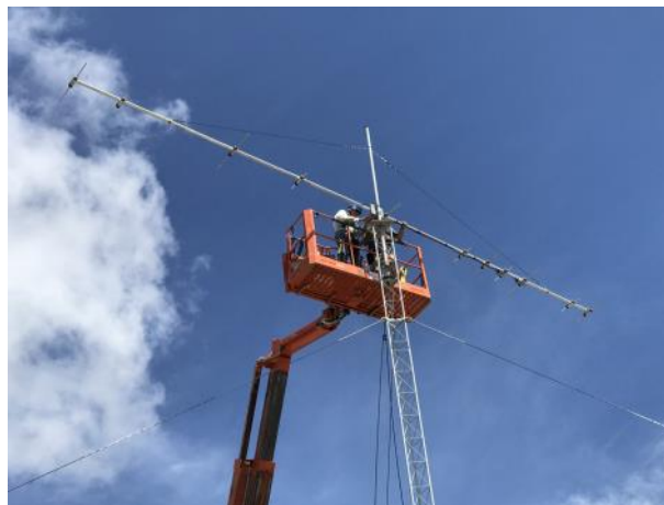
Installing the 1015 36-foot boom
