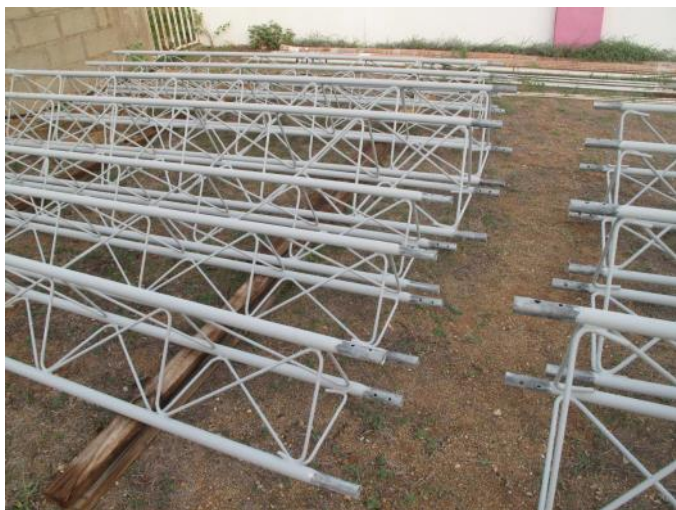
Left: New, painted tower sections Right: Tower top plates and guy brackets
