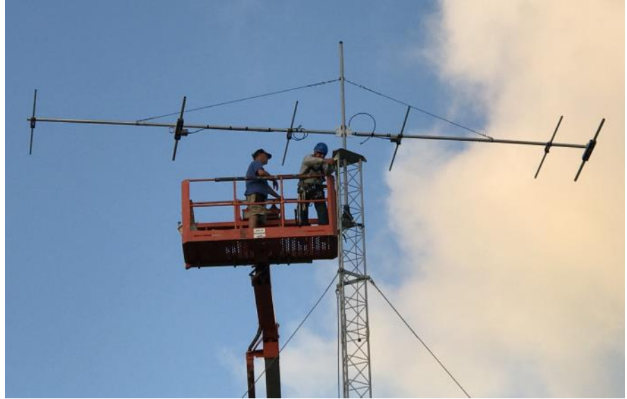
The 2040 boom installed with the centers of the elements
