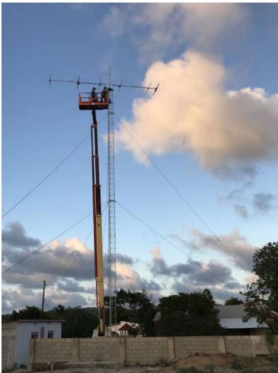
The 2040 being installed on the Rohn 45
