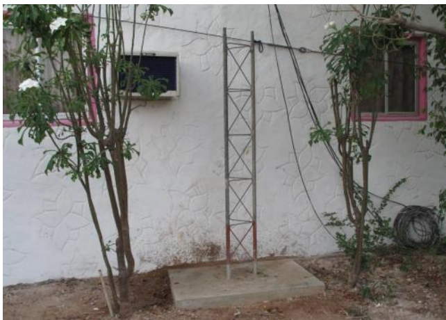
The North Rohn 25 with new base section and concrete installed by JP
