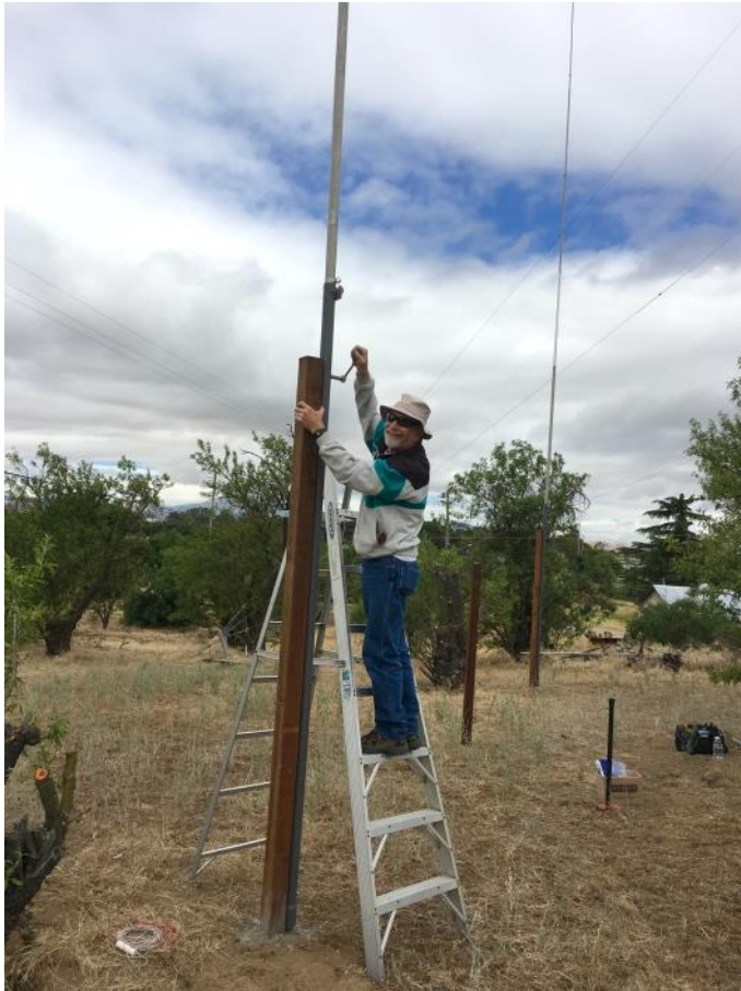
Figure 3. WB6ETY bolts the East element into place.
