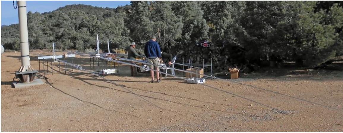
Figure 6 – Final assembly of the version 3 of the 80M elements.
