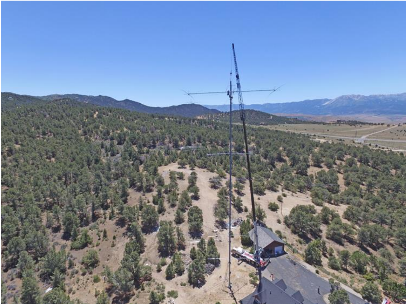
Figure 8 – Finally, XE2K is attaching the new 3 element 80 at the top of the 175' monopole. This photo was taken by AA7XT and his drone.
