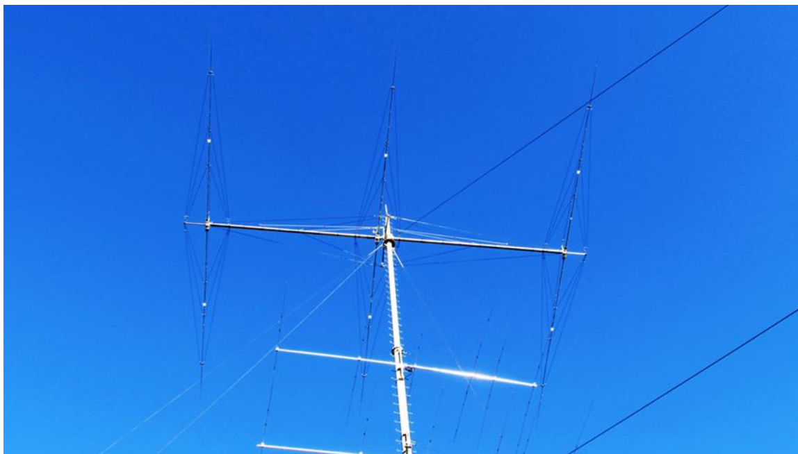
Figure 3 – Super-trussed second erection of the 3 element 80.
