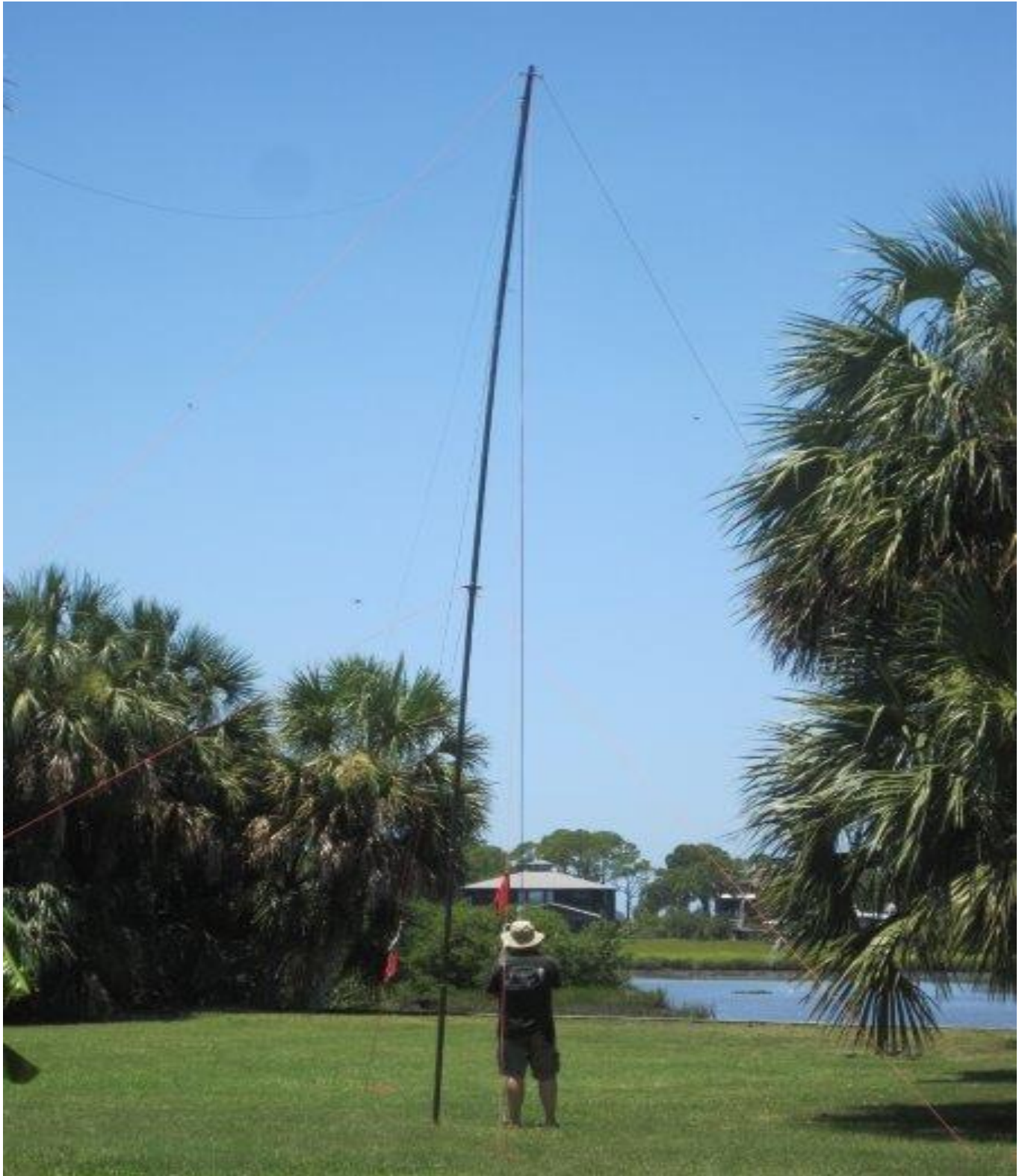
(Setting the guy lines for a 10–80 OCF dipole)
