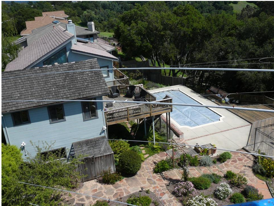
View from the basket at 45 feet up.
