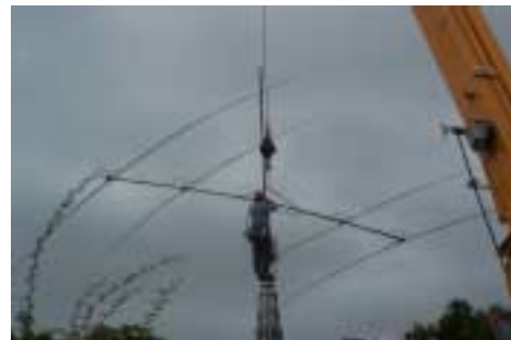
Steve, K7LXC, mounts the EF240/230 to its mast plate.
