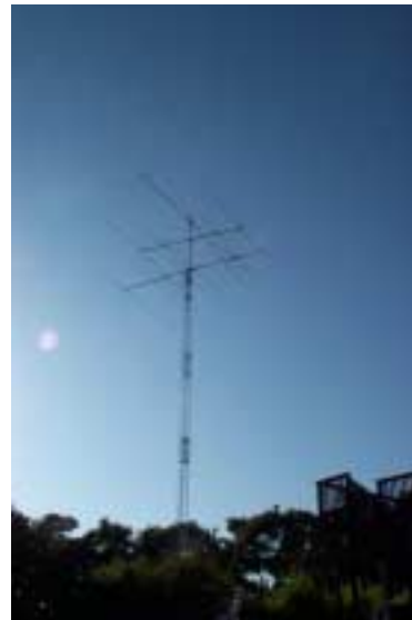
Force 12 5BA, EF240/230 and Sigma 180S on a 72-foot crankup at K6RB.
